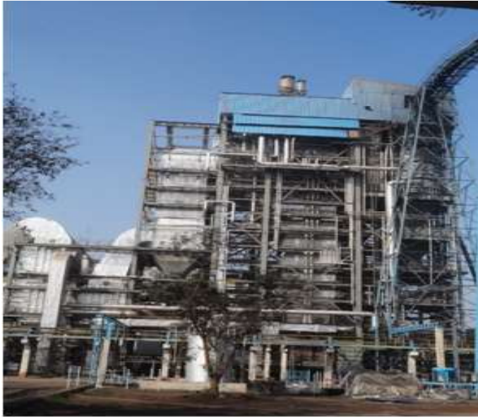
60 MW Captive Power Plant
